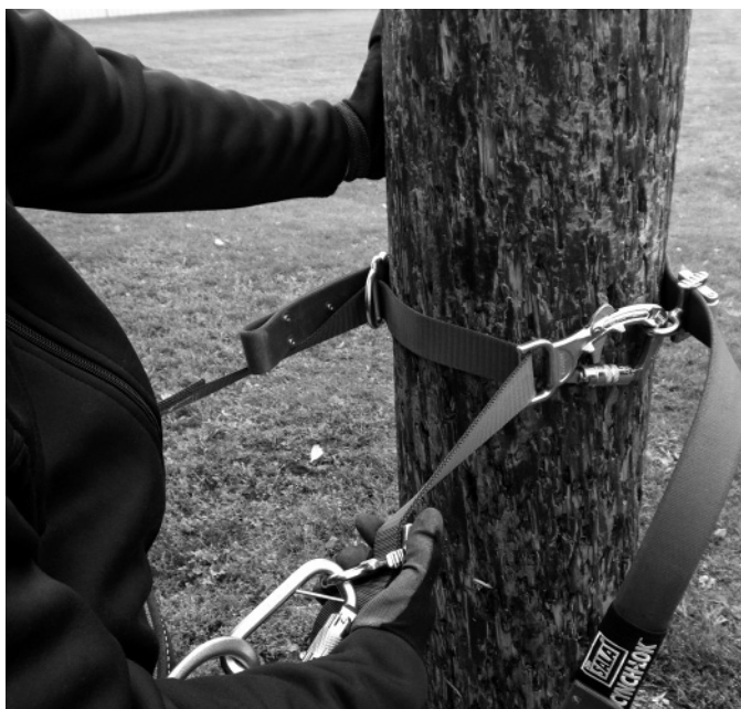
Figure 23 - Adjust Forward into Pole, Web Version
